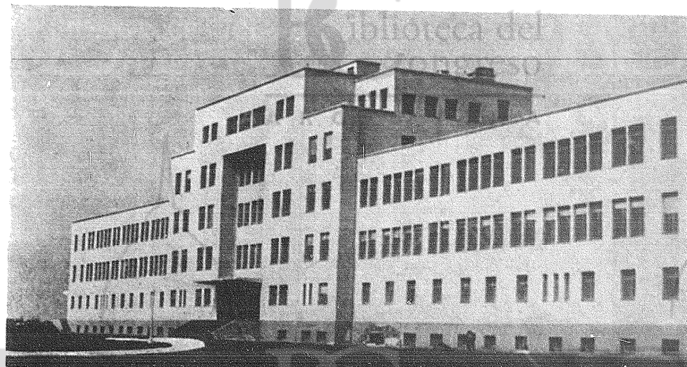
The constructive trade unionism which is practised in Argentina is distinguished for its social work. This polyclinic is the work of the Glassworkers' Union.
